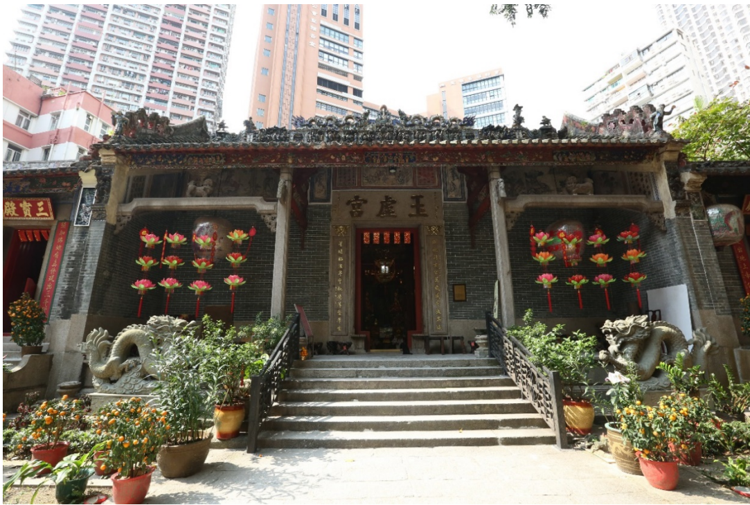
Facade of the main building, with Shiwan ceramic figurines on the ridge made by Junyudian (均玉店) in 1907, and granite architrave with inscribed characters “玉虛宮” written by Zhang Yutang (張玉堂) in 1862
